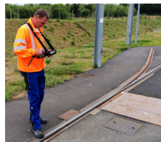
Visual inspection of switch
