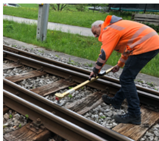
Taking measurements on a switch
